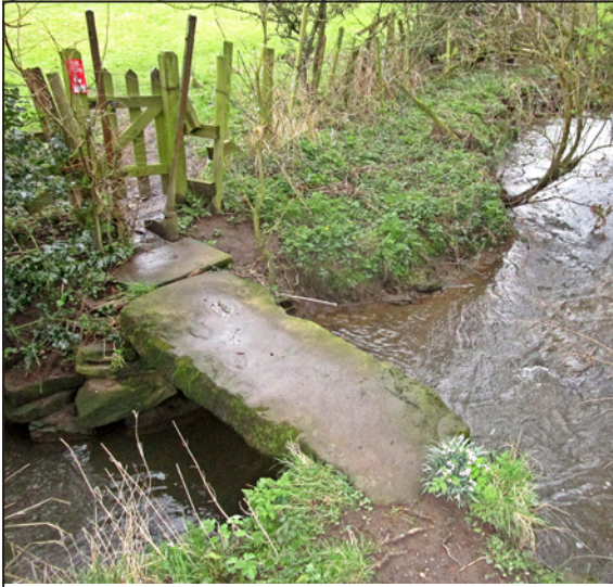
Old stone bridge at Nether Heage.
