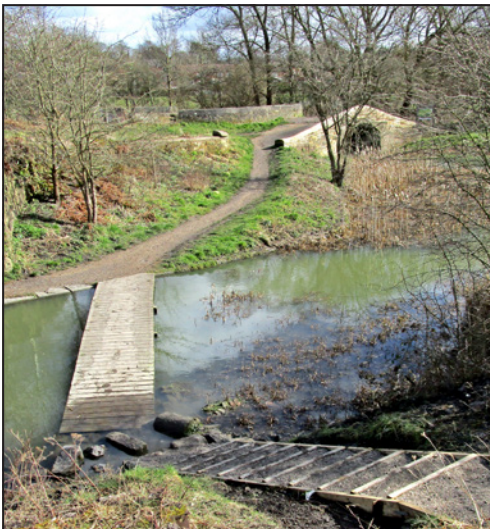
An overview of the lower steps, the boardwalk and 'Humpty' Bridge.
