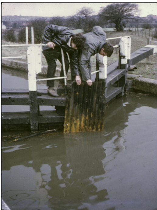
... a sheet of corrugated iron was 'acquired' and used to stem the flow of water between the gates as the lock was emptied. Holidaymakers of today might be a little surprised by the boating techniques of 50 years ago!
