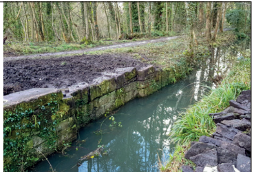
Removal of a large tree root and replacement of the stones revealed the full extent of the recess for one of the gates on the stop 'lock' beside the cottage.
