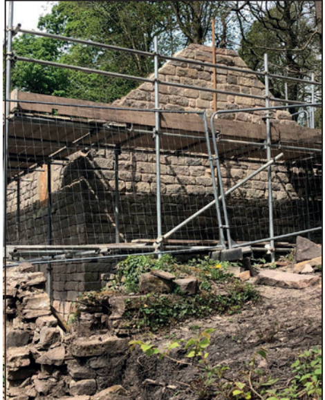
The restored gable end.
