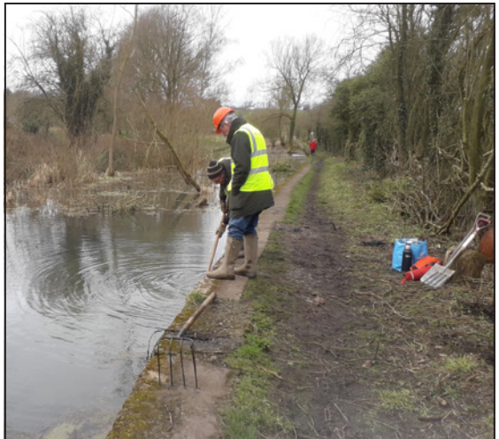
Clearing the blocked culvert at Hartshay.
