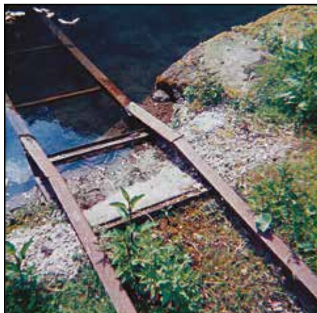
The rails entered the water at the point of the peninsular where boats were launched and recovered.
