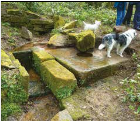
The large stone that is thought to be the base of a crane used to lift stones from road wagons onto boats. The dogs give the scale! The purpose of the stone-lined water channel on the left is a mystery.
