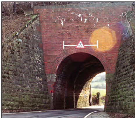
The opposite side was brick faced, possibly because of collapse of the original stone facing.
