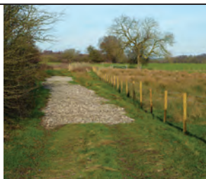
Recent resurfacing of the route near Stoneyford.
