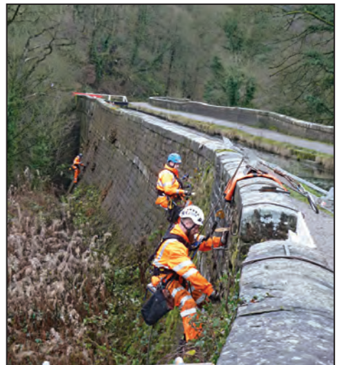
Rope access contractors clear Derwent Aqueduct of unwanted vegetation.
