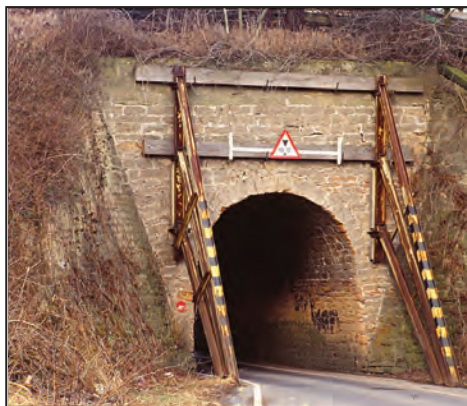
The original stone face of Mill Lane Bridge with supporting beams.
