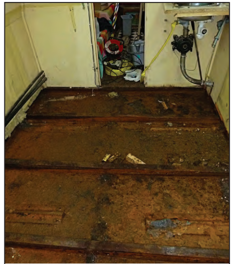
And finally cleared, awaiting a coat of red oxide, and reassembly.
