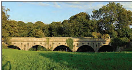
The M&PR's 1819 Portland Viaduct is the oldest railway viaduct in England.
