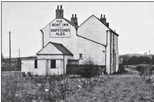
The Boat Inn at Pinxton was the terminus for the first passenger journeys on the M&PR. This view, probably from the 1950s, shows the canal well overgrown if not infilled. The canal here has since been rewatered, along with the terminal basin, and whilst the structure of the Inn still stands it has been greatly extended and was scheduled to reopen in late November.
