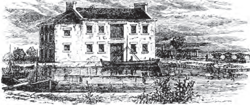
The warehouse at Pinxton with the clerk's office at the end was built by the M&PR in 1817. After the decline in canal traffic it was used for concerts, magic lantern shows, boxing etc and was named Palmerston House. At one time it became a public house known as the Palmerston Arms.
