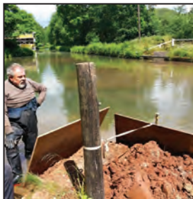
Puddling the leak at Leawood sluice.
