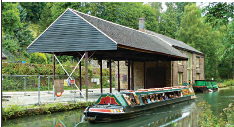
The canopy adjacent to the Wharf Shed before and after work had been carried out. Note the cross-bracing that has been added. At the end of August it was awaiting a final coat of paint on the metalwork. Photos: Hugh Potter
