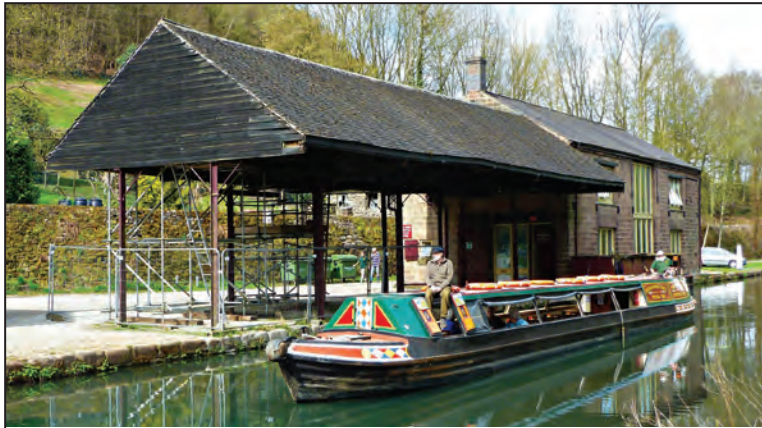
The canopy adjacent to the Wharf Shed before and after work had been carried out. Note the cross-bracing that has been added. At the end of August it was awaiting a final coat of paint on the metalwork. Photos: Hugh Potter
