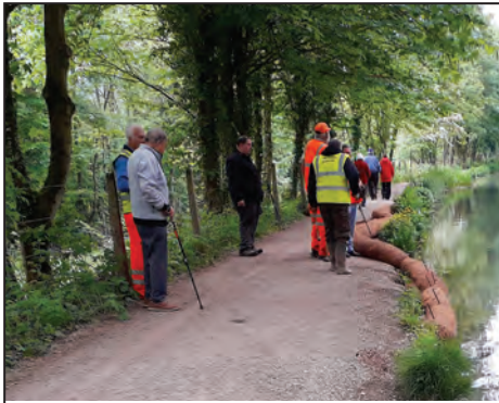
Manoeuvring a giant coir sausage into place. Photo: John Guyler
