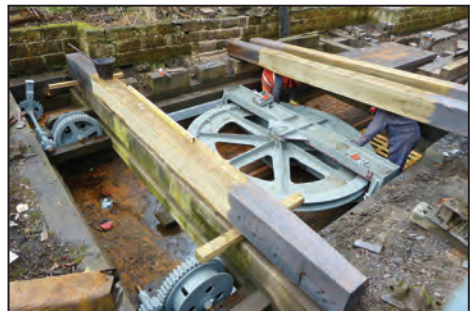
Replacement of the incline pulley wheel underway at High Peak Junction. Photo: Editor
