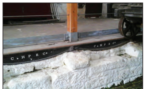
Fish-bellied rail as originally used on the CHPR, possibly the oldest railway line in the world still in its original location.
