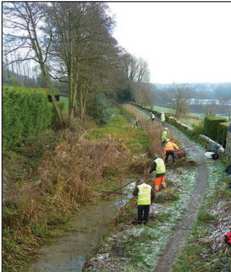
What a difference a day makes . . . the view from Poyser's Bridge at Ambergate as work began and after completion. Water could once again flow through the formerly reed-blocked channel where there was no access for machinery.
