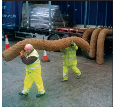
Unloading coir rolls from the oversize truck at Cromford Wharf.
