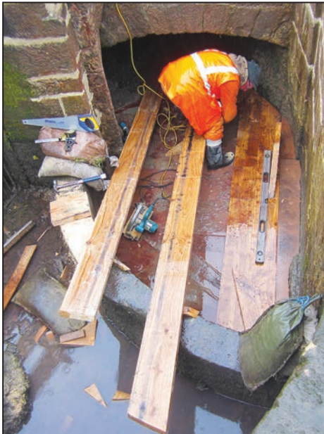
New oak boarding being fitted.
