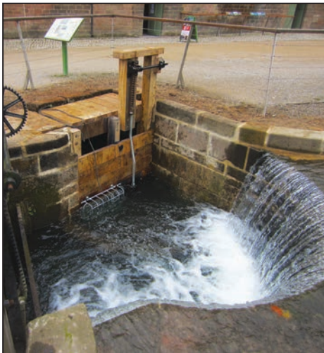
Water starts flowing again to the canal.
