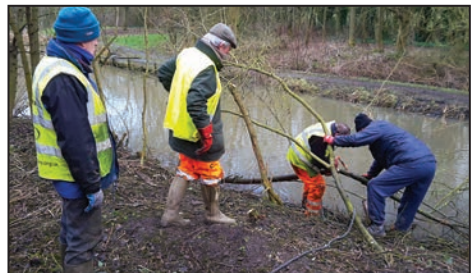
Clearance work at Pinxton Wharf. Photo: John Guyler
