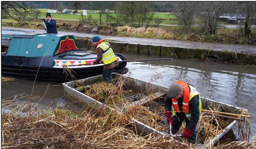
Reed pulling at Lawn Bridge in January.
