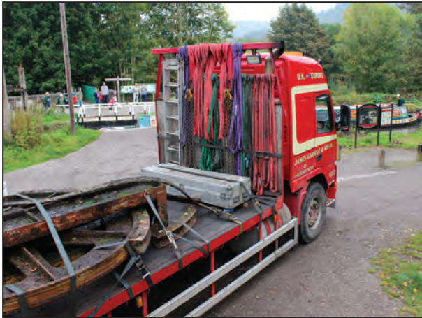
The partly deconstructed CHPR pulley wheel about to be taken for restoration as Birdswood passes through the adjacent swing bridge. Photo: Rick Jillings
