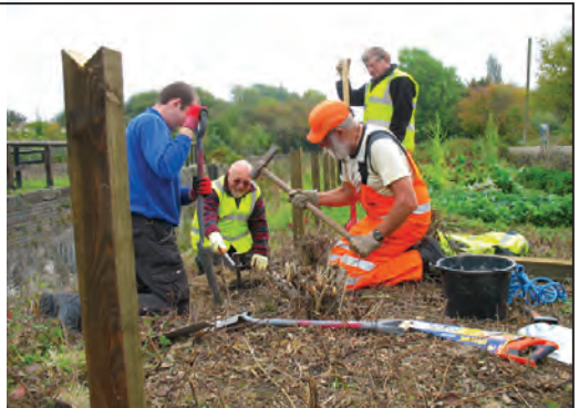
Installing safety fencing around the garden at Lock 4.
