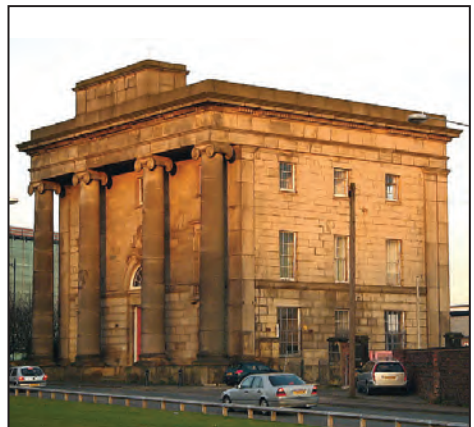
Curzon Street Station, Birmingham, was built with stone carried on the Cromford Canal.
