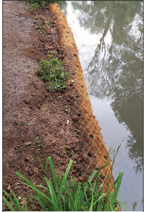
. . . and backfilled with clay, awaiting the original vegetation to be replaced.
