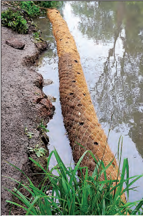
The coir roll in place . . .
