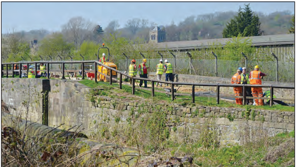
The view of work from across Lock 4. Photo: Pete Clark
