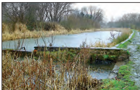
Plenty of water both in the canal and on the towpath at the site of the dam placed across the canal by the Butterley Co to ensure sufficient water supply for their forges when they used to operate close to the canal here below Lock 7.
