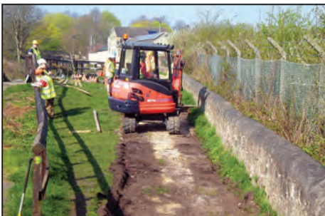
The old surface was removed with a mini-digger.
