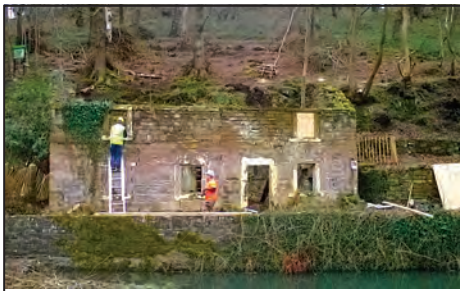
Work underway on the cottage.
