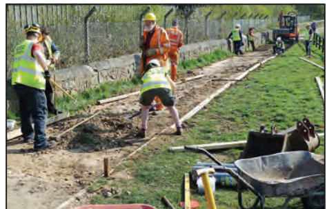
Laying the hardcore on the Terram liner.
