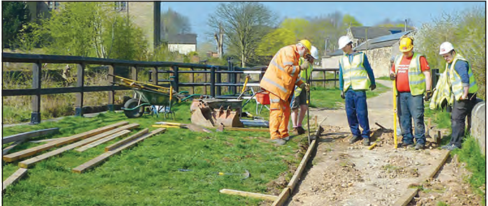
Plenty of supervision setting up the shuttering.
