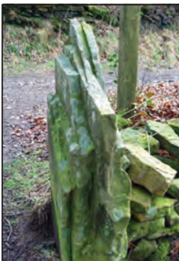
This stile post on Hearthstone Lane shows the raw ‘stone slate’ material that was available in the area to the south-east of Riber.
