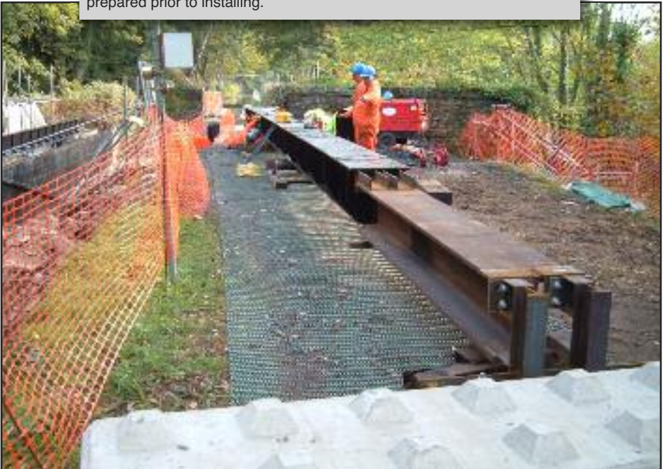
ABOVE: When the welding was completed, the whole structure was cleaned and painted inside and out. BELOW: One of the two beams which will support the new towpath being prepared prior to installing.
