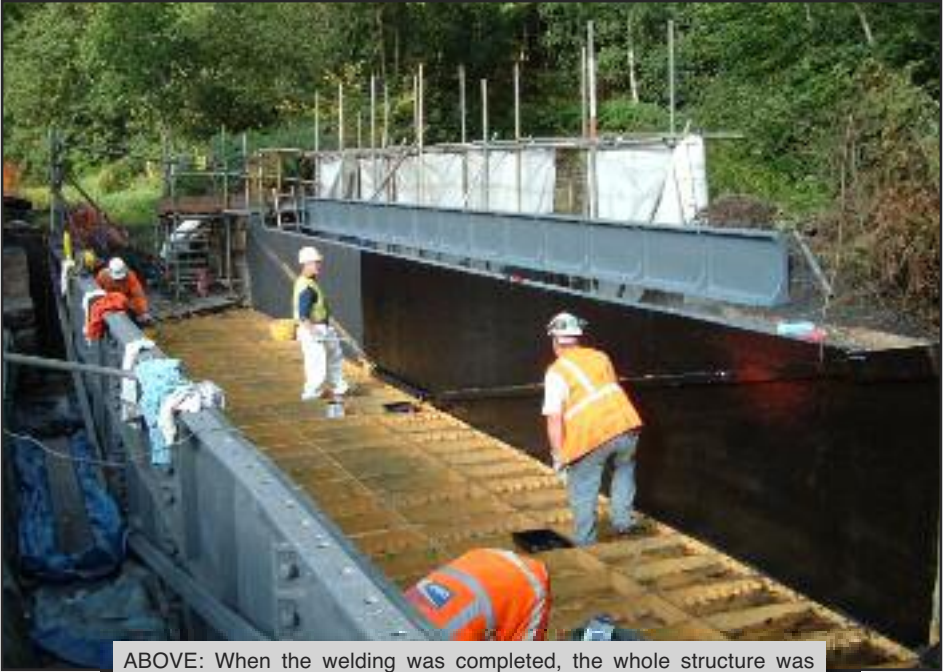
ABOVE: When the welding was completed, the whole structure was cleaned and painted inside and out. BELOW: One of the two beams which will support the new towpath being prepared prior to installing.
