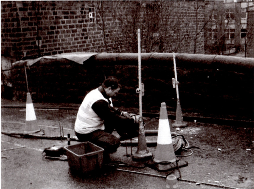
Injecting the Grout
