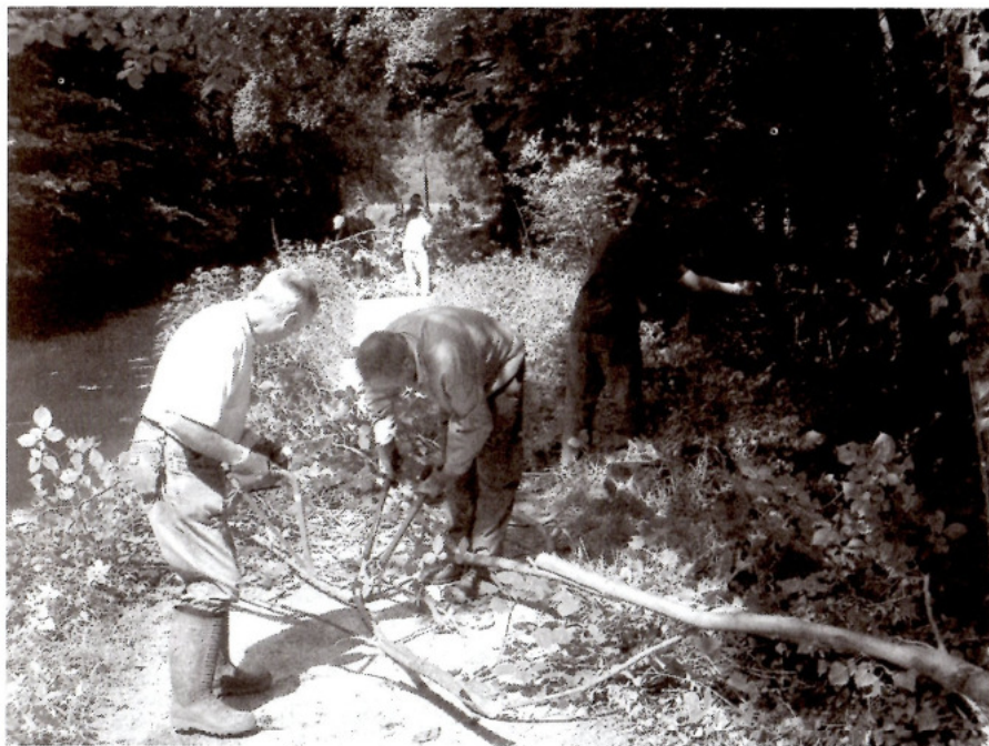
Cutting away the overgrowth
