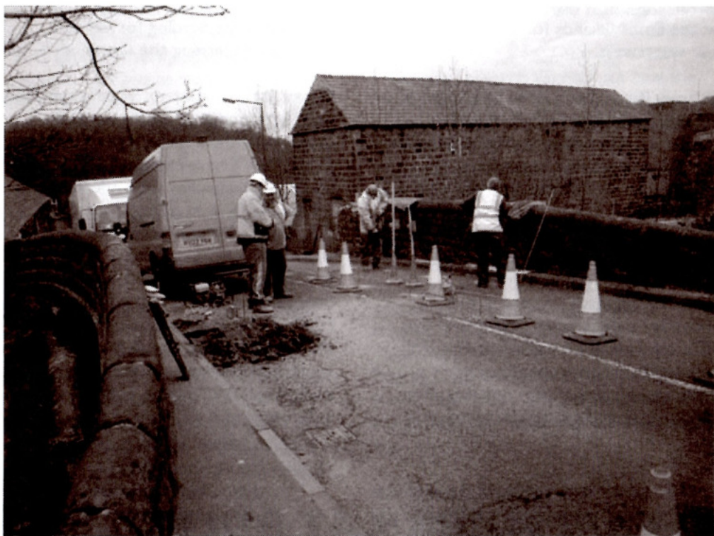
Preparing to inject the grout
