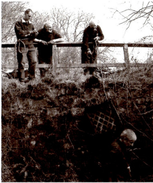
The end of March saw us at Ironville locks, shifting rubbish.....
