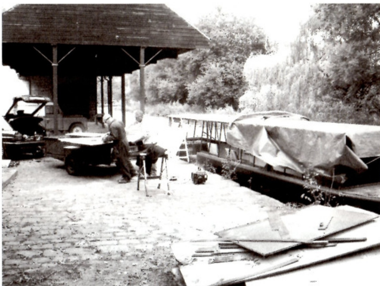
The new roof's going on nicely.....
