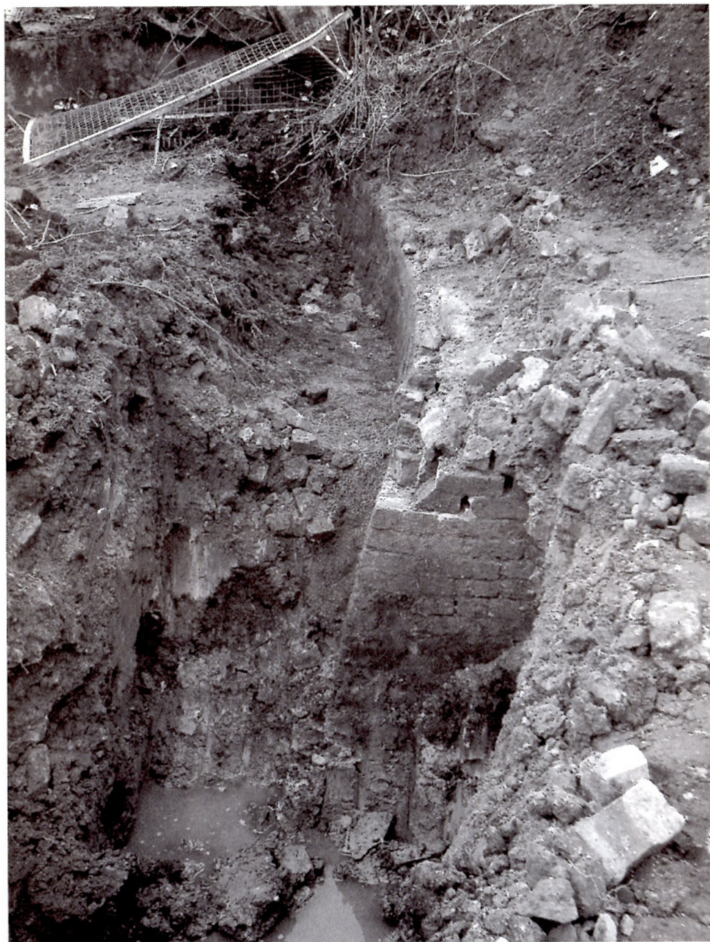
So that's what it's all about. The north-east wing wall curving towards the camera and the remains of the bridge arch running from left to right.
