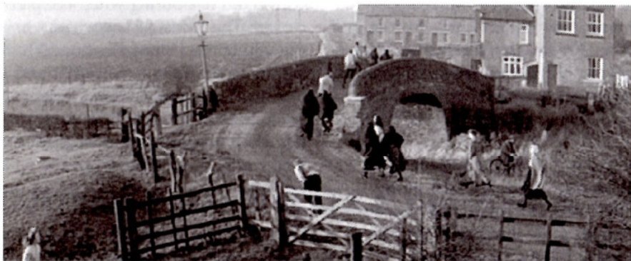
A still from Sons & Lovers, showing the bridge in question
