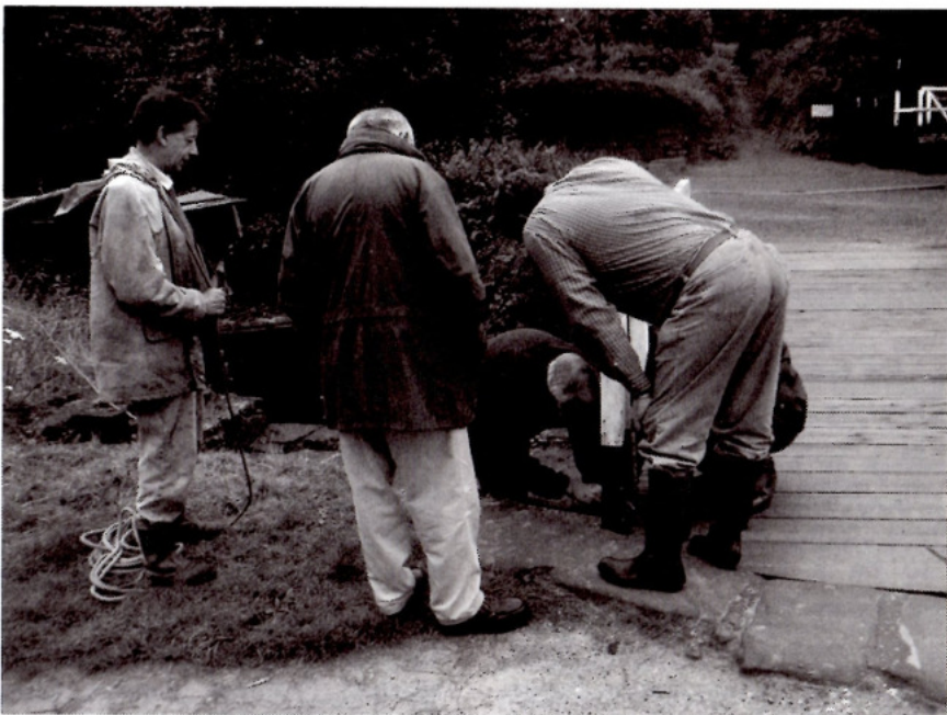
The FCC Technical Committee working on the swing bridge
