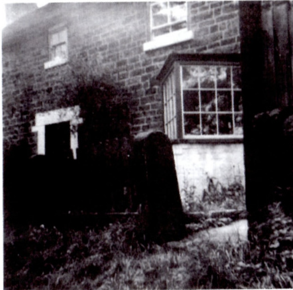
The view of 'Canal House' at Sawmills from the towpath, showing the distinctive triangular bay window which would have enabled the toll keeper to keep a watch for approaching traffic.
