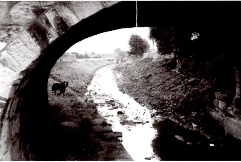
The 'landscaped' channel below Bridge 37 looking down to Lock 4.
