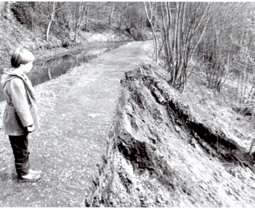
25 th February 1989 immediately on the morning the canal overtopped. Approx 200 yards East of iron aqueduct. Small boy is my son, David. Only the new steel piling installed in late 1988 prevented a complete disaster.
