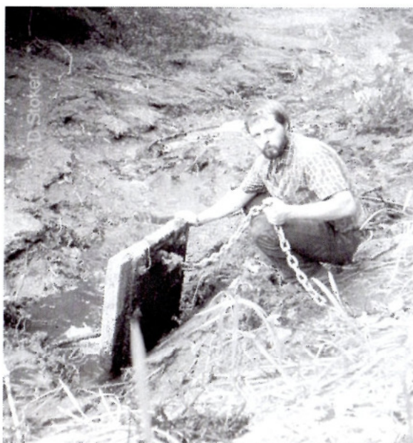
One of the trapdoors set in the bed of the canal. About halfway between Cromford and High Peak. The person is a young Simon Stoker.
