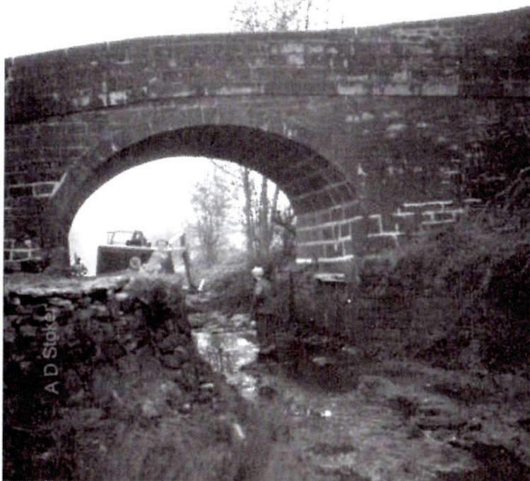
The result of having cleared through the bidge.
