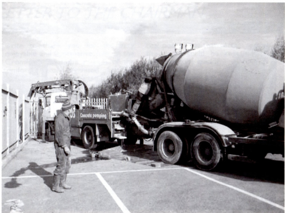
Pumping the concrete.....
