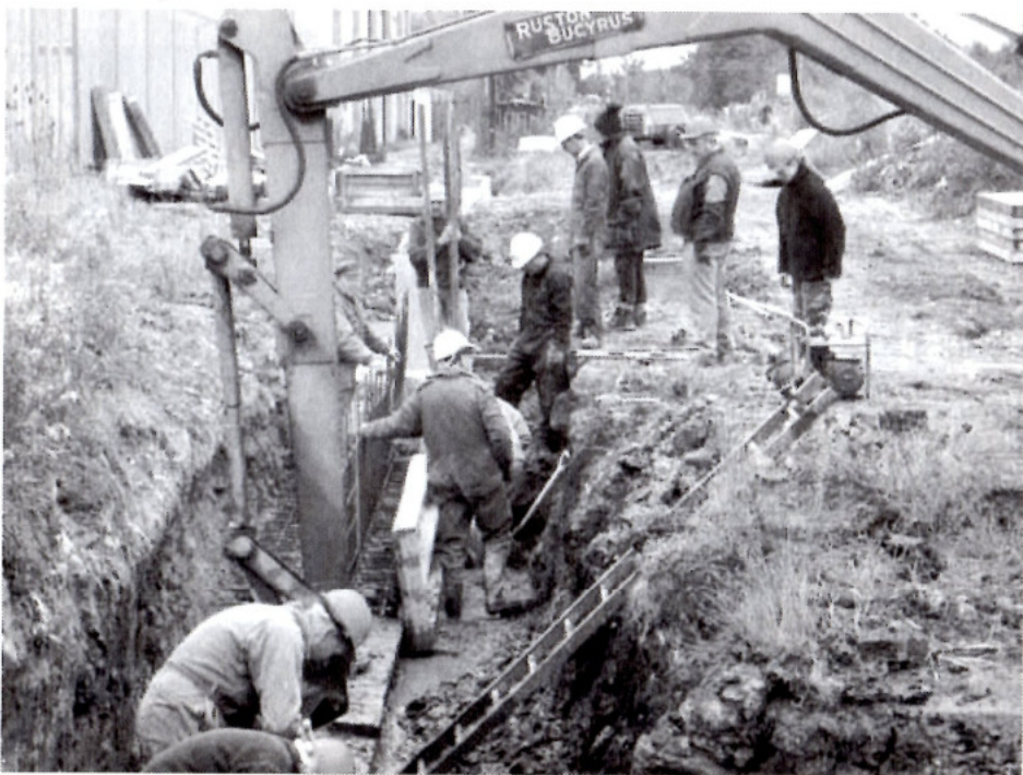
The shuttering in place.....
