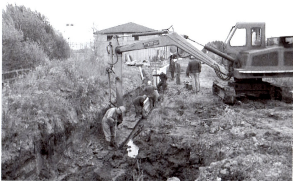
The wall exposed.....
