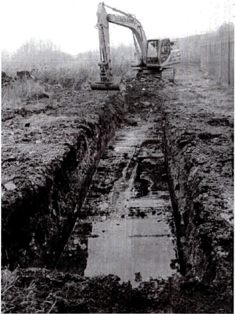
"Hey lads - we've found a canal wall in trench one!" (As Tony Robinson would say on "Time Team" (The Editor) )
